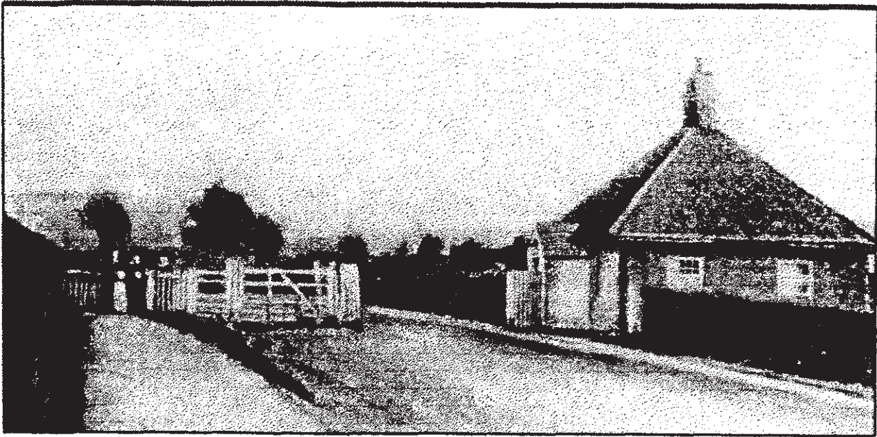
Reproduction from a painting, looking South, by the father of the late Mr. E.J. ("Mayor") Holt from Houghton Regis. This old toll house and gate was situated at the Kenworth side of Half Moon Hill, on Watling street. It was demolished around 1880. It was certainly very similar to the Puddle-Hill Toll-Gate House and Cottage of the article.
