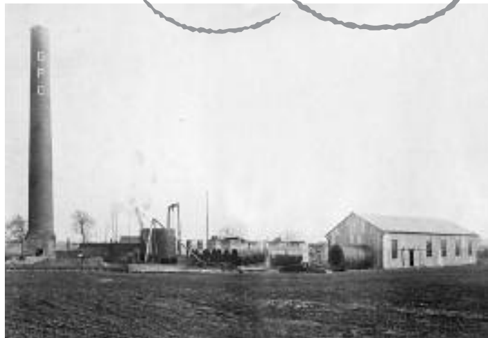
The cement works being constructed at Houghton Regis in November 1925
