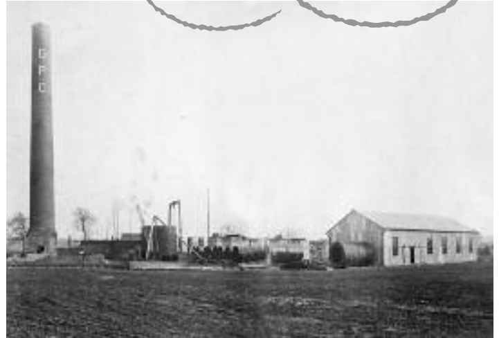
The cement works being constructed at Houghton Regis in November 1925
