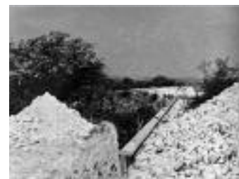
Chalk Hill slurry bridge, 1969
