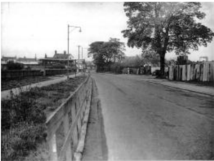
The construction of the Empire Rubber Company in London Road during 1938
