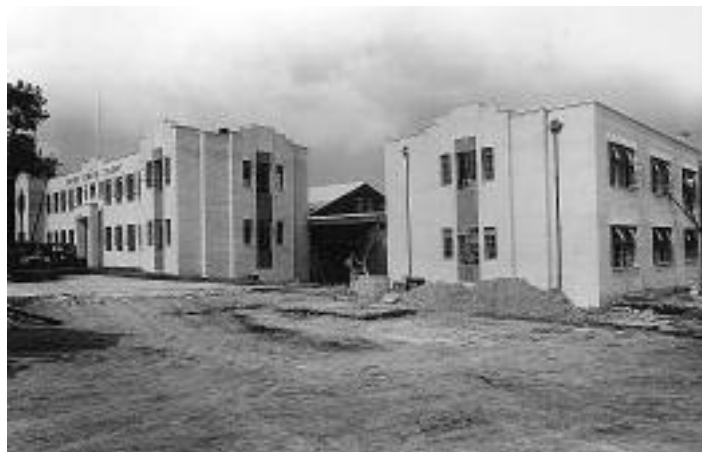
The construction of the Empire Rubber Company in London Road during 1938
