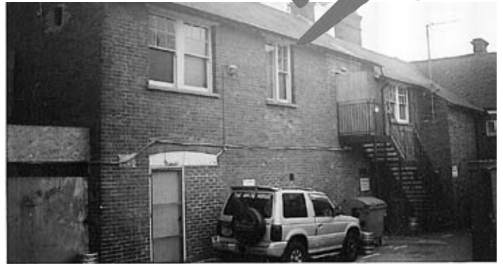
Dart factory site rear of Anchor archway
