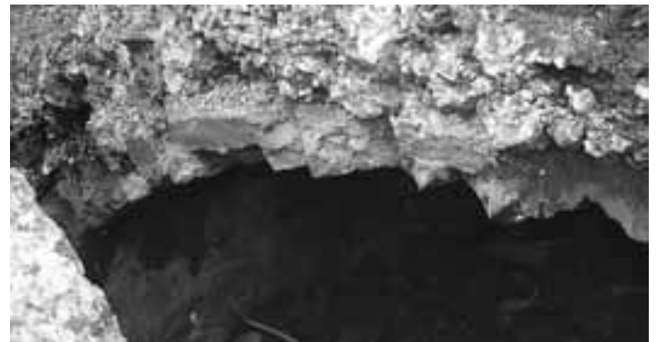
The top of the domed brickwork with the cavity beneath
