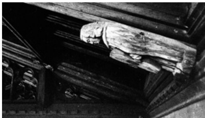
One of the roof figures showing the rafters
