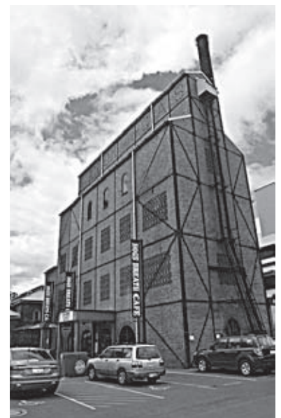
The building in Launceston, Tasmania which bears an amazing resemblance to one in the Dunstable Goods Yard
