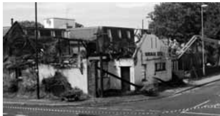
The remnants of the Norman King after the fire
